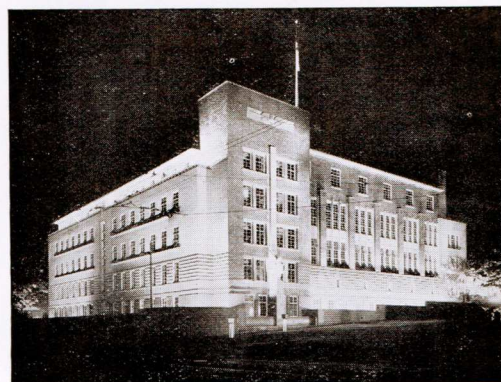
Administrative Offices, Bristol Aeroplane Co. Ltd.
